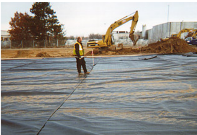
Application of a base stabilization woven slit-film geotextile
