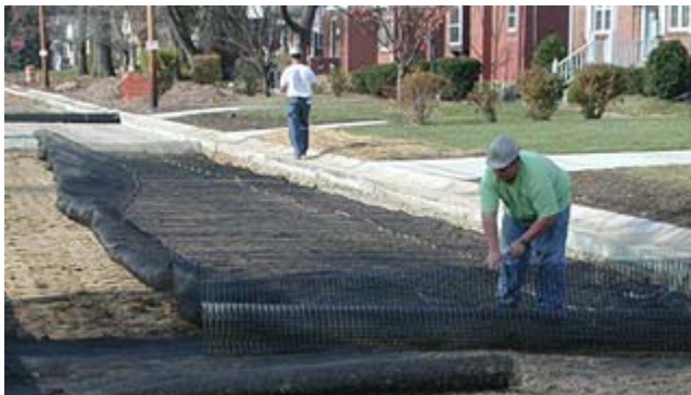
Application of a base stabilization geogrid
